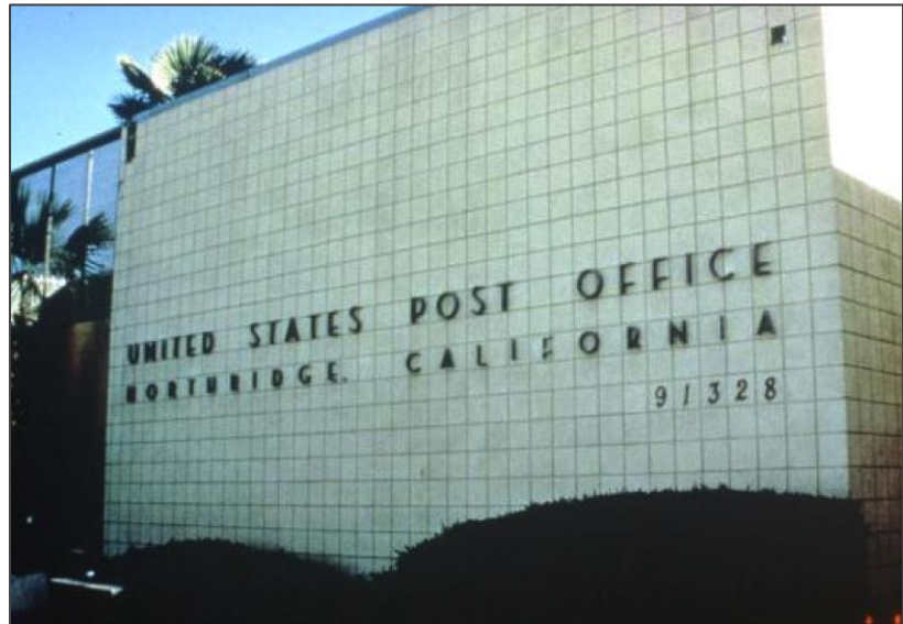
Reinforced Block Structure
