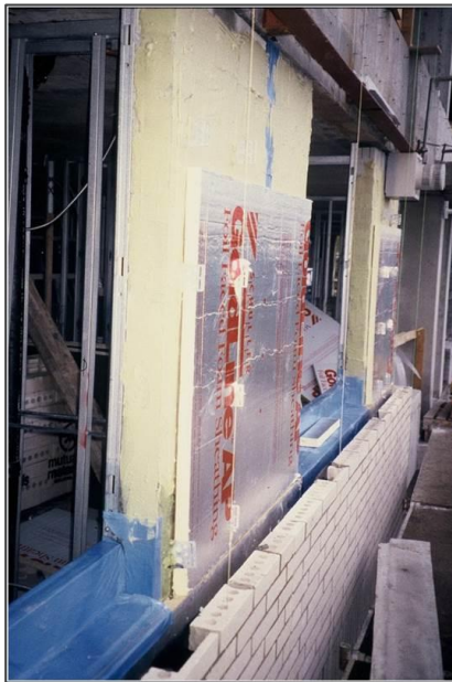
Elm Park Place – Brick Veneer over Block Backup
